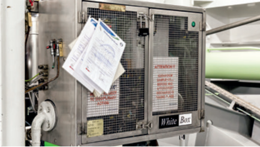
The White Box is where all the monitoring and control values for the bilge water are recorded. It is secured with a separate lock to protect the data against manipulation from outside.
